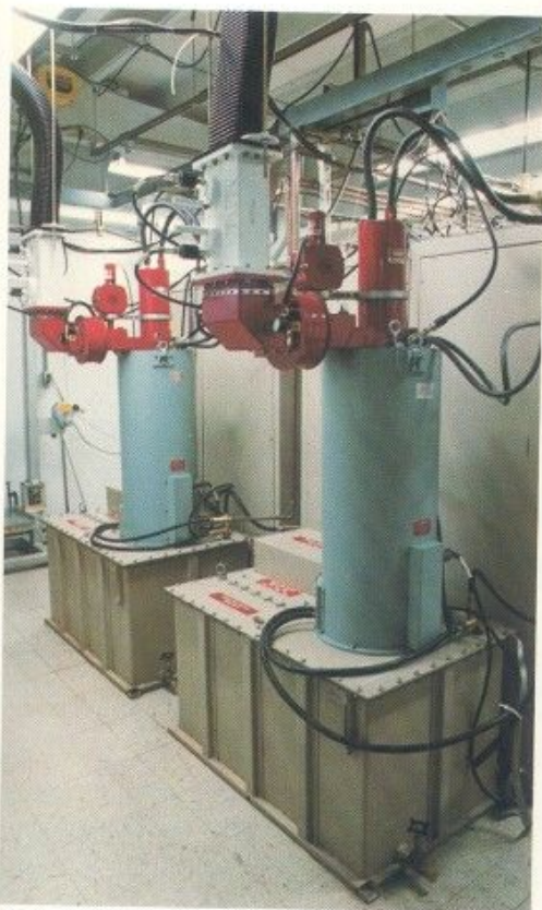
These dual klystron amplifiers have an operational life of from three to four years.
