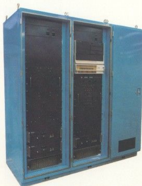
The TCCS links controllers with each other and with all communications circuits including air-to-ground radios.
