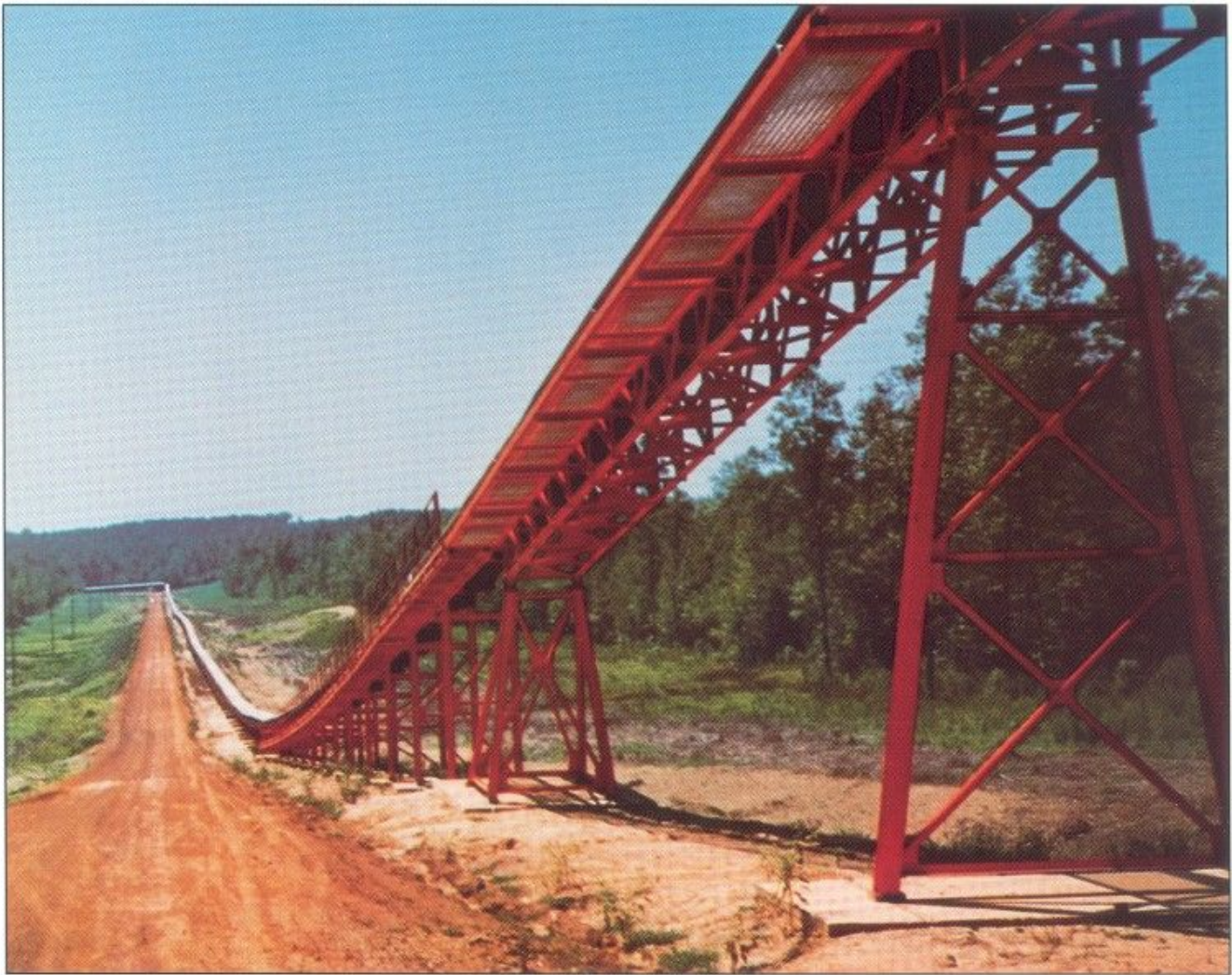
A 7-mile-long overland Continental conveyor carries 14,000 to 15,000 tons of lignite daily.
