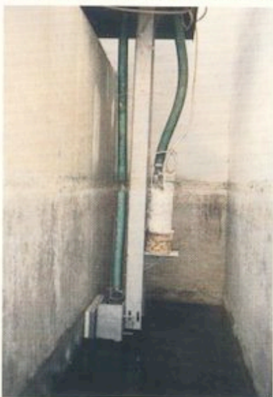
Conventional TBF problem #6—bridge derailment caused by side load on bridge from sliding shoe
