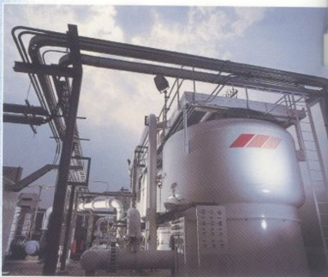
BOC Gases' vacuum swing adsorption (VSA) plants are ideal for providing oxygen for small to medium furnaces.
