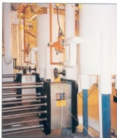
A Welded plate heat exchanger cools propylene glycol at Nestle USA, Inc. Modesto, California plant.
