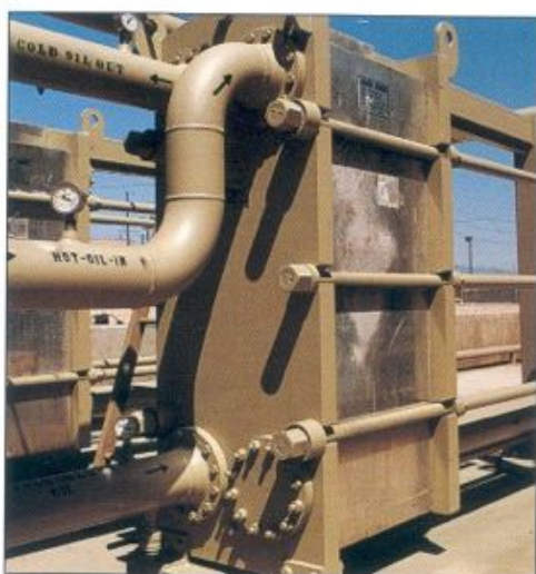
Two PHEs handle heavy crude oil water at Union Oil, California.
