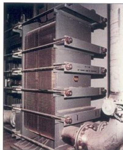
Reinforcements or "dog bones" are indicative of obsolete plate heat exchanger designs.
