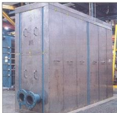
For protection on light hydrocarbon services, Alfa Laval's fire shroud withstands temperatures up to 1500°F.
