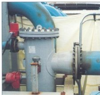
Alfa Laval's automatic back flushing strainer protects plate heat exchangers from debris.
