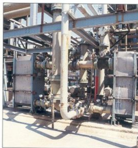
Two PHEs cool dilute sulfuric acid (1-3%) from a scrubbing tower with cooling tower water at Big River Zinc, Sauget, Illinois.
