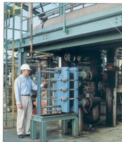
A Diabon F® PHE cools a mixture of hydrochloric acid and chlorinated hydrocarbons, Union Camp, Florida.
