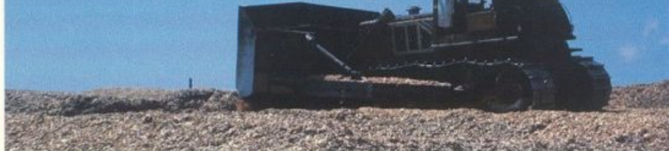
Bulldozers damage chips as they run over the wood pile. Automated chip handling systems eliminate this problem, saving money through conservation of usable fiber.
